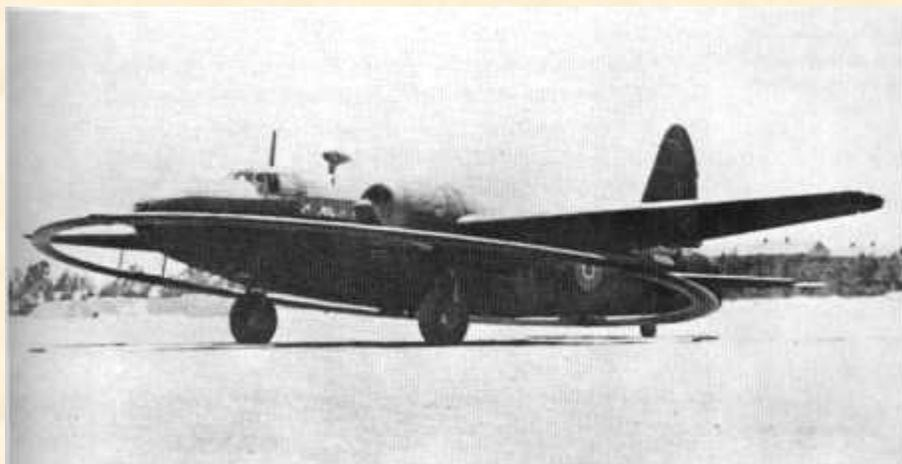
The DWI Wellington before take-off. Despite the coil, the plane was reported to handle extremely well in flight.
